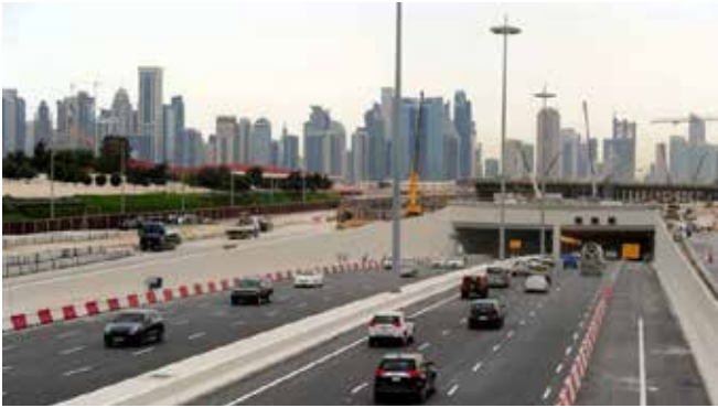
LUSAIL CITY, TUNNEL VENTILATION, QATAR
